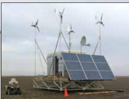
The Point Barrow shore station runs on wind and solar energy to power the radar in a remote setting.
